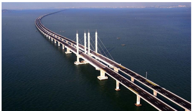
跨海大桥 by Forsandy01
